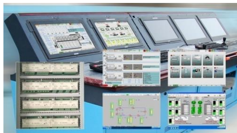
Cabin microcomputer alarm monitoring system
